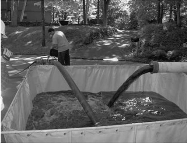
FIGURE 20-17 Effluent from a pigging operation showing slurry of accumulated manganese deposits causing hydraulic impairment and black water episodes.
