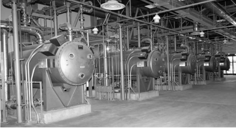
FIGURE 7-6 Illustrative picture of an ozone generator facility. (Photo courtesy of Jim Kostelecky, Metropolitan Water District of Southern California.)
