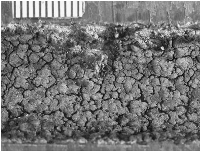
FIGURE 20-15 Lead service line specimen coated with complex material mainly consisting of aluminum, iron, and manganese mixed with phosphate, causing problems with erratic lead release and ineffectiveness of orthophosphate treatment. (USEPA photo.)
