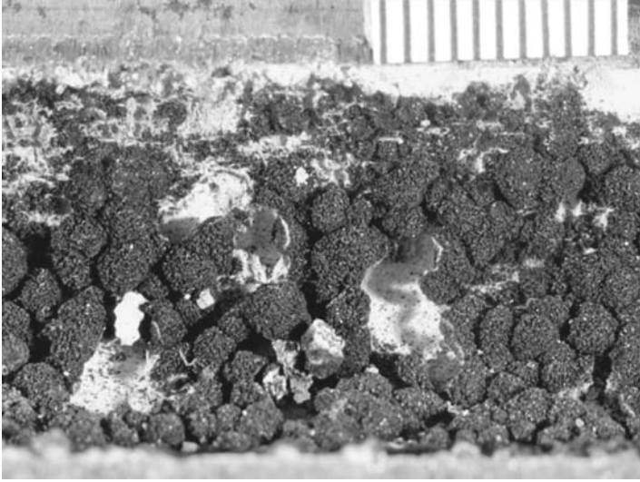
FIGURE 20-16 Lead service line with mainly manganese oxyhydroxide coating on top of normal lead carbonate, resulting in erratic lead release and prolonging the time necessary for passivation and conversion to hydrocerussite in the lead scale. (USEPA Photo.)
