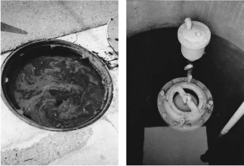
FIGURE 21-13 Photographs of flooded air-release and air-vacuum vaults (the vault on the right contains a dead mouse). (Source: LeChevallier et al., 2002.)
